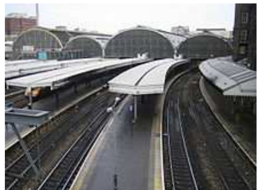
View of the four arches of the station roof
